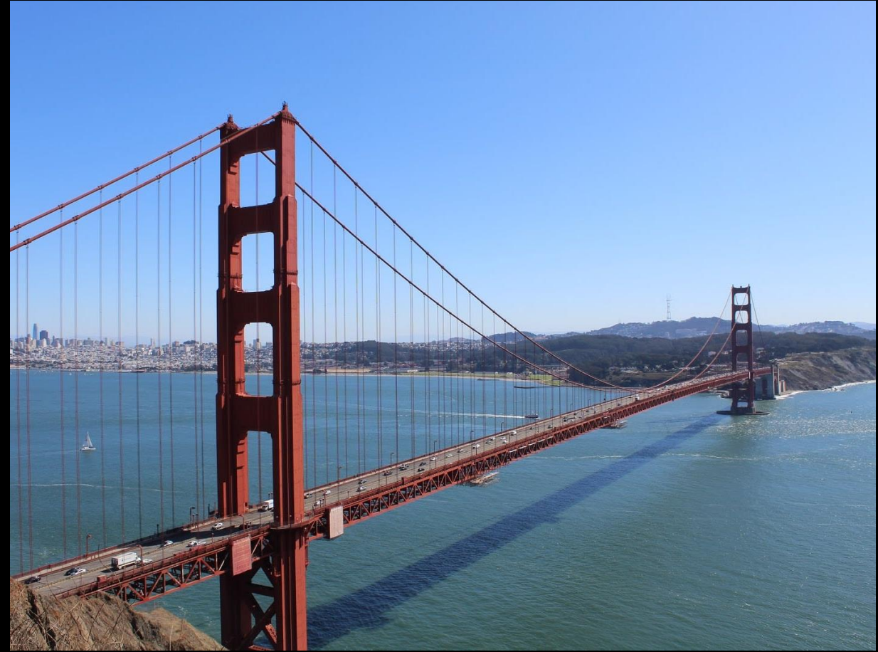
Golden Gate Bridge, San Francisco
